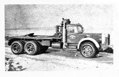
"fifth wheel." By a quick adjustment, the coupler can be raised and the truck used as a tractor to haul oilfield trailers or floats. A "live roll" loading device is installed on the rear of the deck to facilitate loading and unloading the 25 to 30 ton loads that are quite common.
